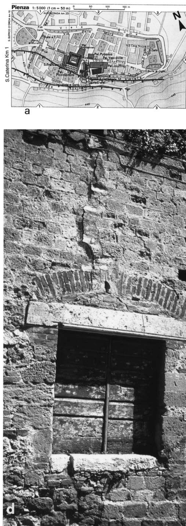
Fig. 25 - a. Map of Pienza, where the trend of the fault and the damaged buildings are indicated (the asterisk indicates the lesions of Fig. 25d). b. Particular of the dislocation of the apse with respect to the transept. c. Map of the lesions occurring inside the Cathedral d. Particular of the lesion present in one house of Pienza, near the Cathedral..
